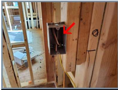
Receptacle rough wiring.
