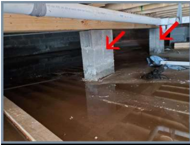
Block piers in crawlspace.
