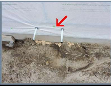
Outdoor shower rough plumbing.
