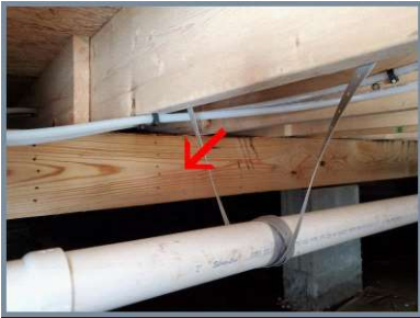
Main beam in crawlspace
