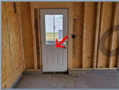
Garage service door.
