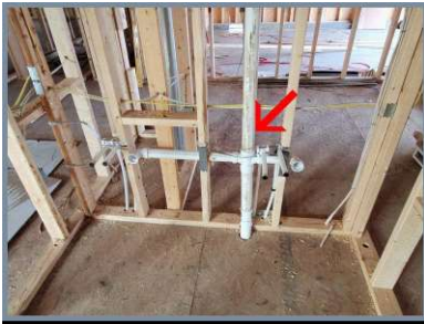
Bathroom rough plumbing.
