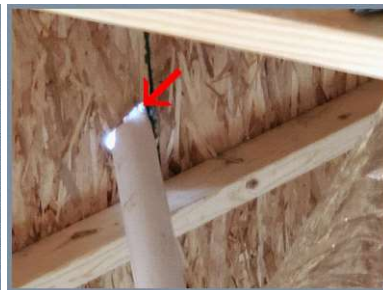
Open interior roof penetration.
