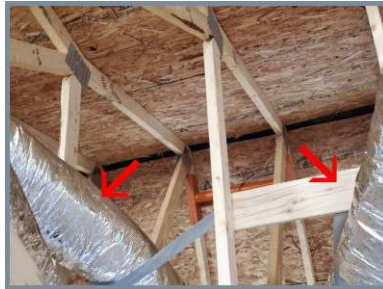
Flexible round supply ducts.
