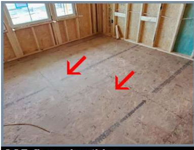
OSB floor sheathing.
