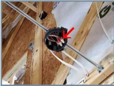
Rough wiring for smoke detectors.
